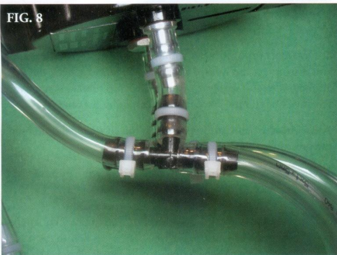
Connections sealed with tie-wraps.
