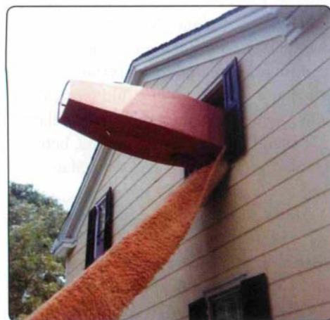
Duster in attic window ready to be lowered.
